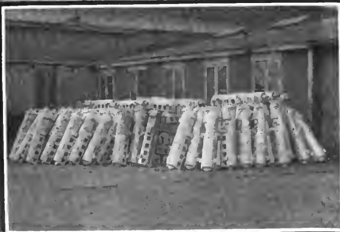
One Day's Foundry Output of Aluminum Crank- cases.
